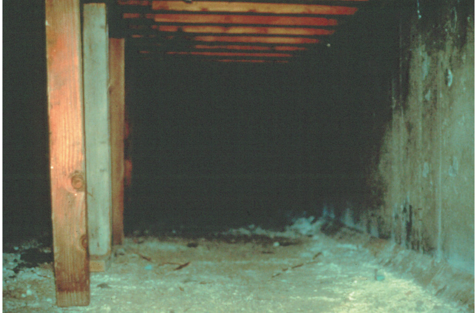
Figure 7.11.37 Interior Formwork Left in Place
