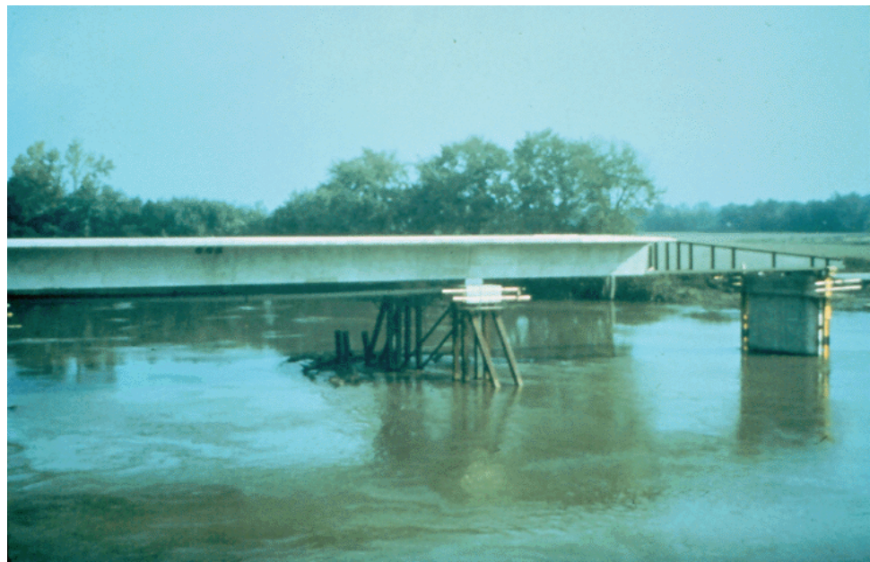
Figure 7.11.25 Incremental Launching Overview (Note Temporary Pile Bent)
