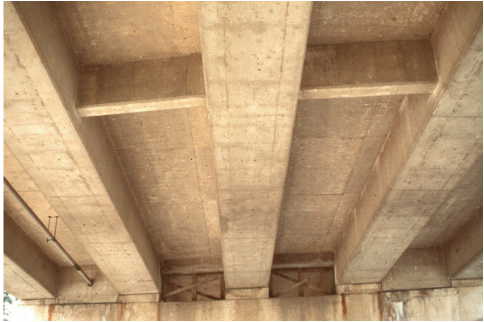
Figure 7.10.8 End and Intermediate Diaphragms on a Spread Box Beam Bridge
