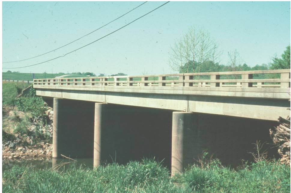
Figure 7.10.1 Typical Box Beam Bridge
