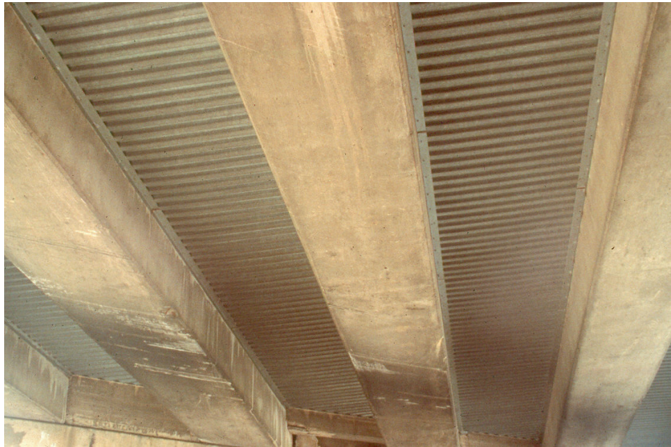
Figure 7.10.7 Underside of a Typical Spread Box Beam
