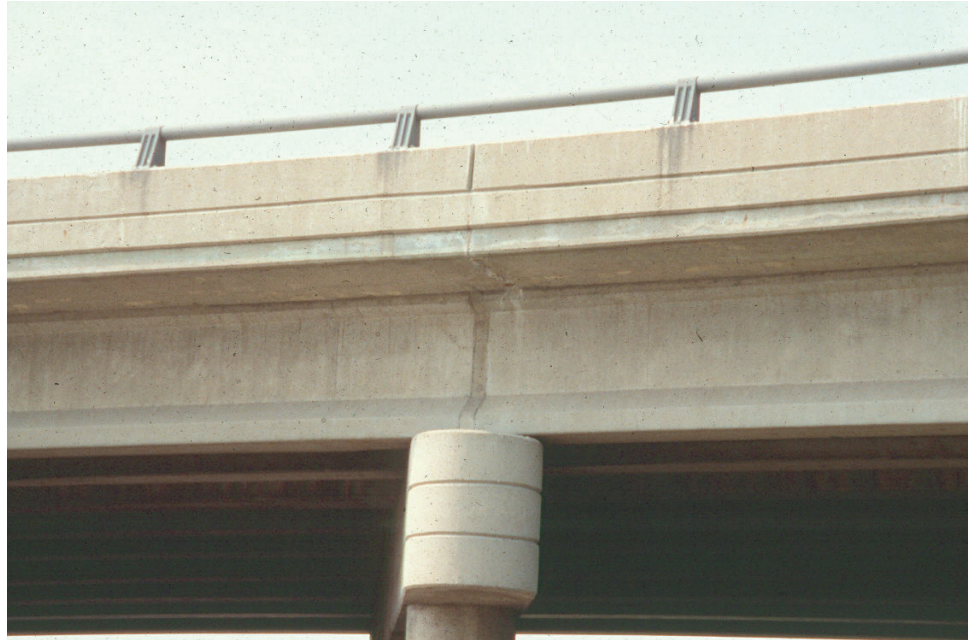
Figure 7.9.5 Continuous Prestressed I-Beam Bridge
