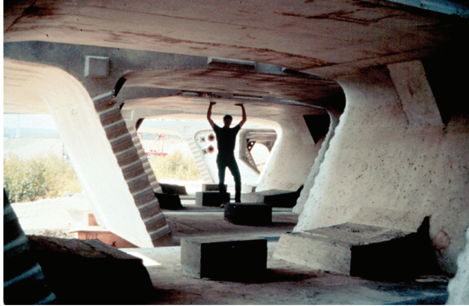
Figure 7.11.16 Box Girder Segment
