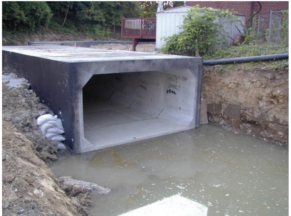
Figure 7.12.4 Precast Concrete Box Culvert
