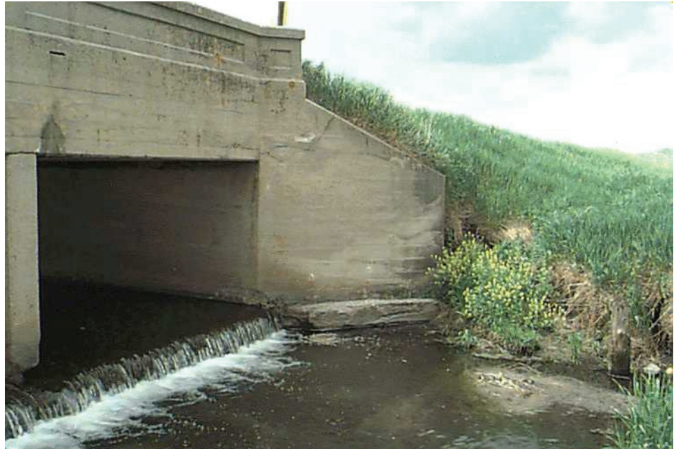
Figure 7.12.9 Cast in Place Concrete Box Culvert Outlet
