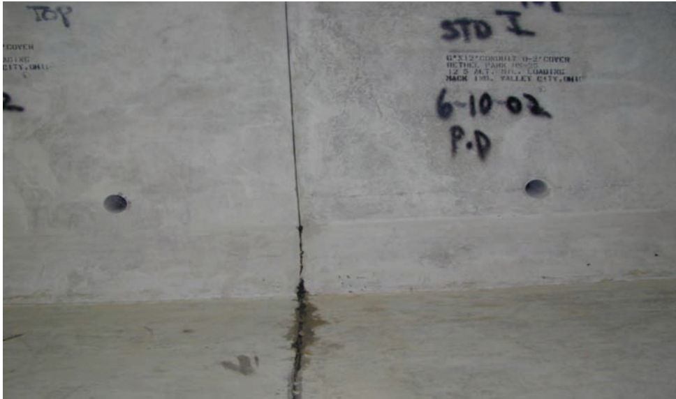
Figure 7.12.8 Precast Concrete Box Culvert Joint
