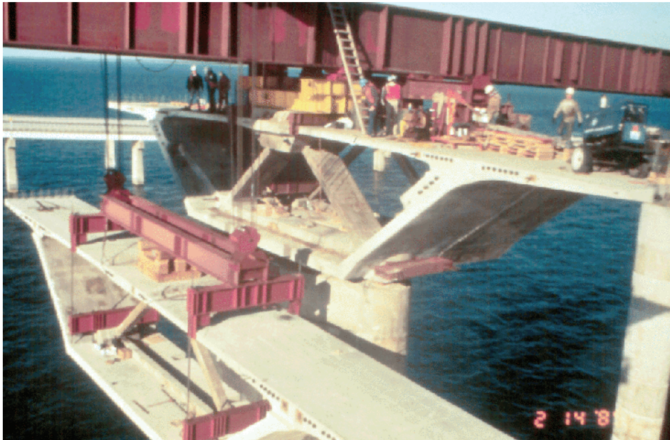
Figure 7.11.18 Balanced Cantilever Construction
