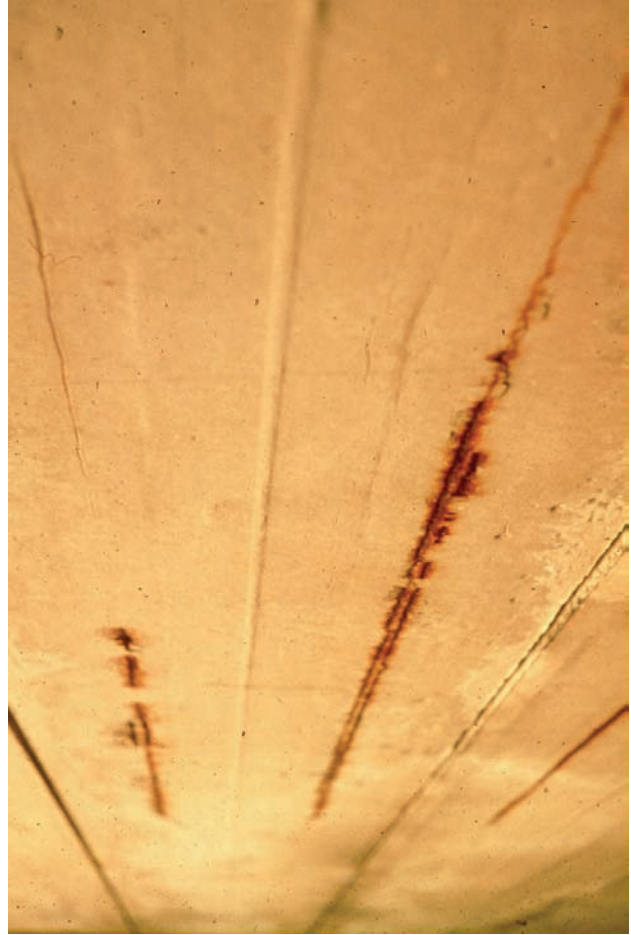
Figure 7.10.18 Burlap Fold Depressions in an Early 1950's P/S Box Beam
