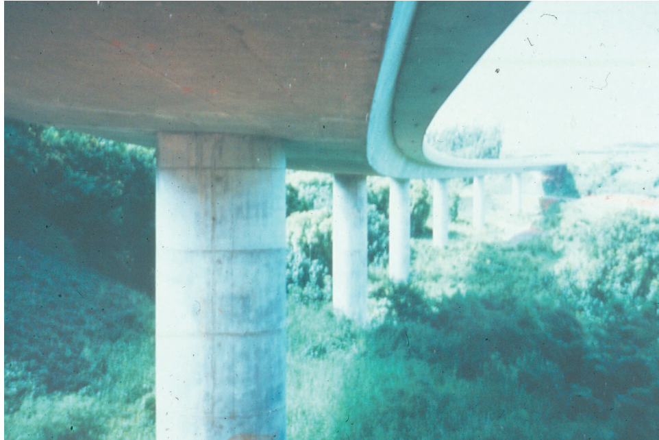
Figure 7.11.2 Cast-in-place Concrete Box Girder Bridge
