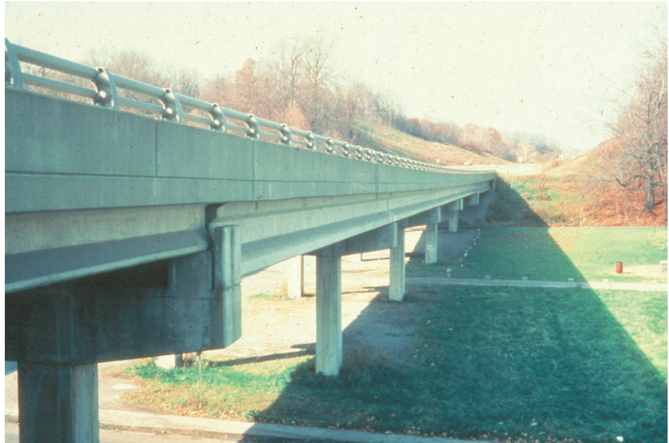
Figure 7.9.1 Prestressed I-beam Superstructure
