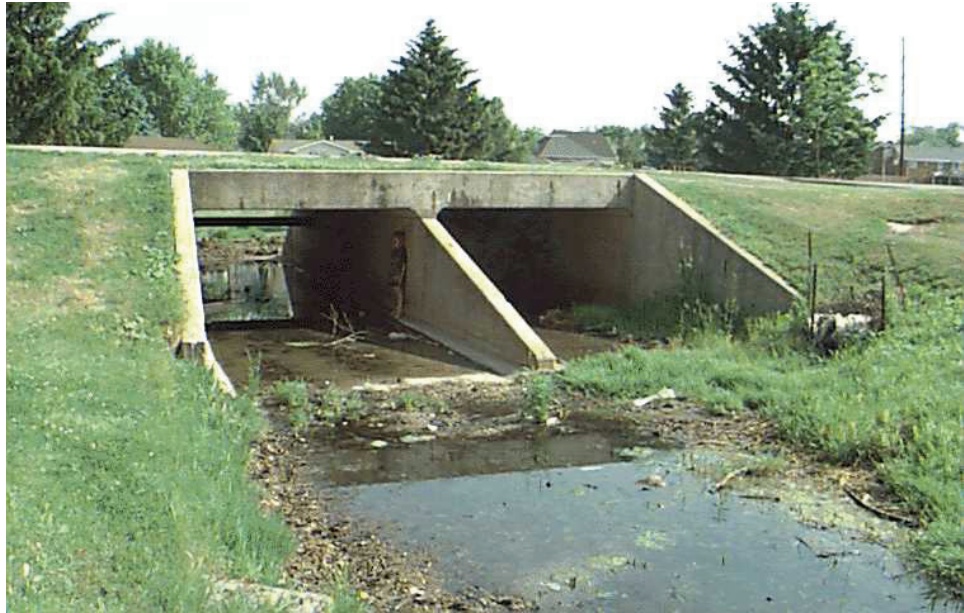
Figure 7.12.2 Multi-cell Concrete Box Culvert
