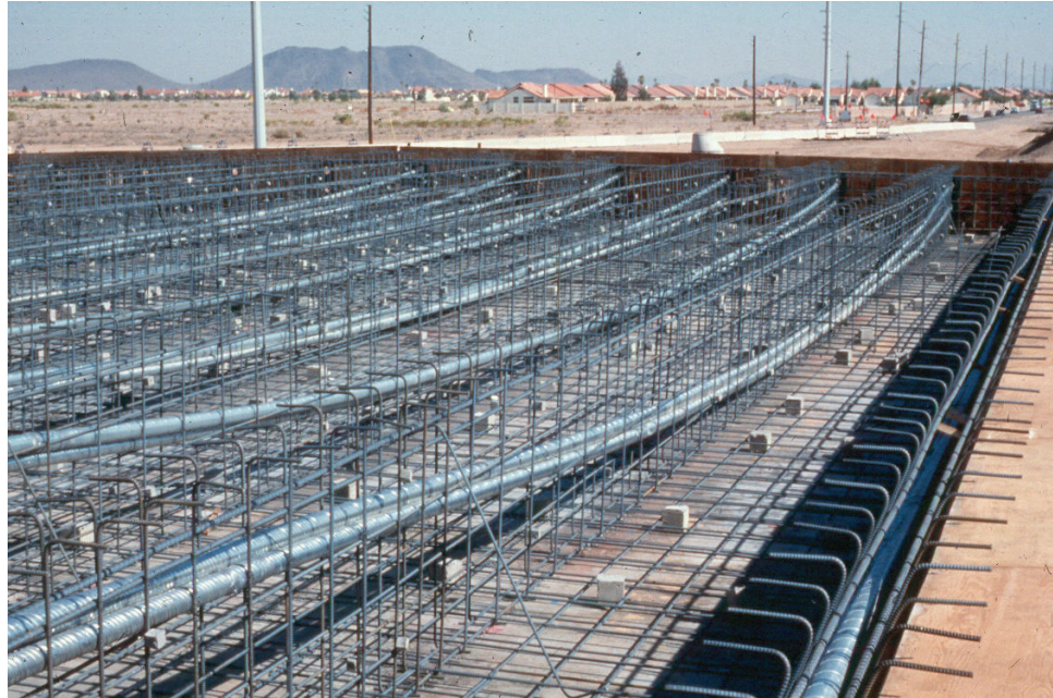
Figure 7.11.6 At-grade Formwork with Post-tensioning Ducts
