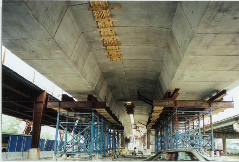
Figure 7.11.12 Adjacent Single Cell Boxes with Closure Pour
