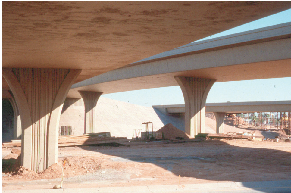
Figure 7.11.7 Box Girder Bridge Construction
