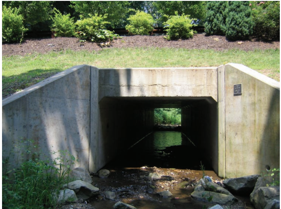
Figure 7.12.1 Concrete Box Culvert
