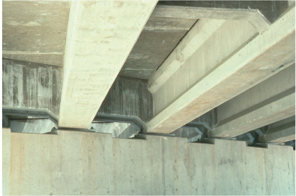
Figure 7.9.7 Concrete End Diaphragm
