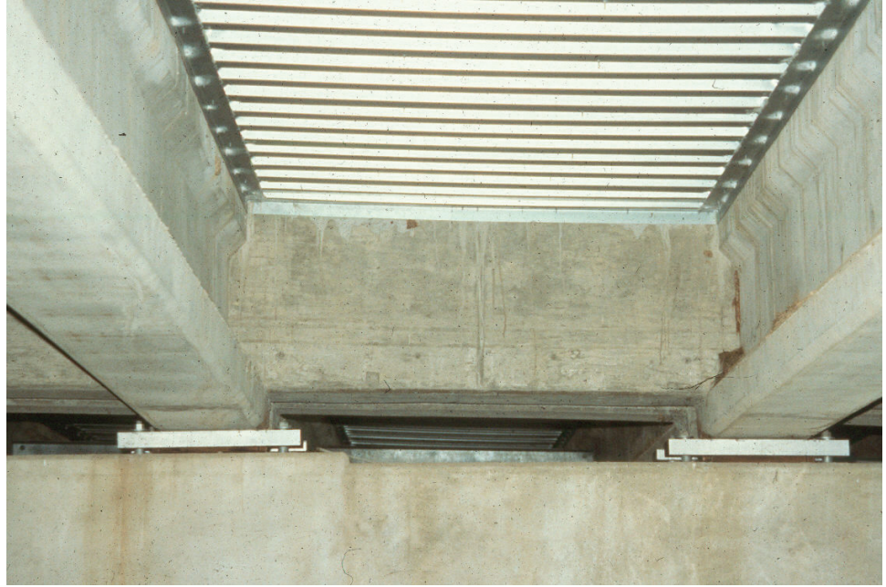
Figure 7.9.12 Typical Concrete Diaphragm
