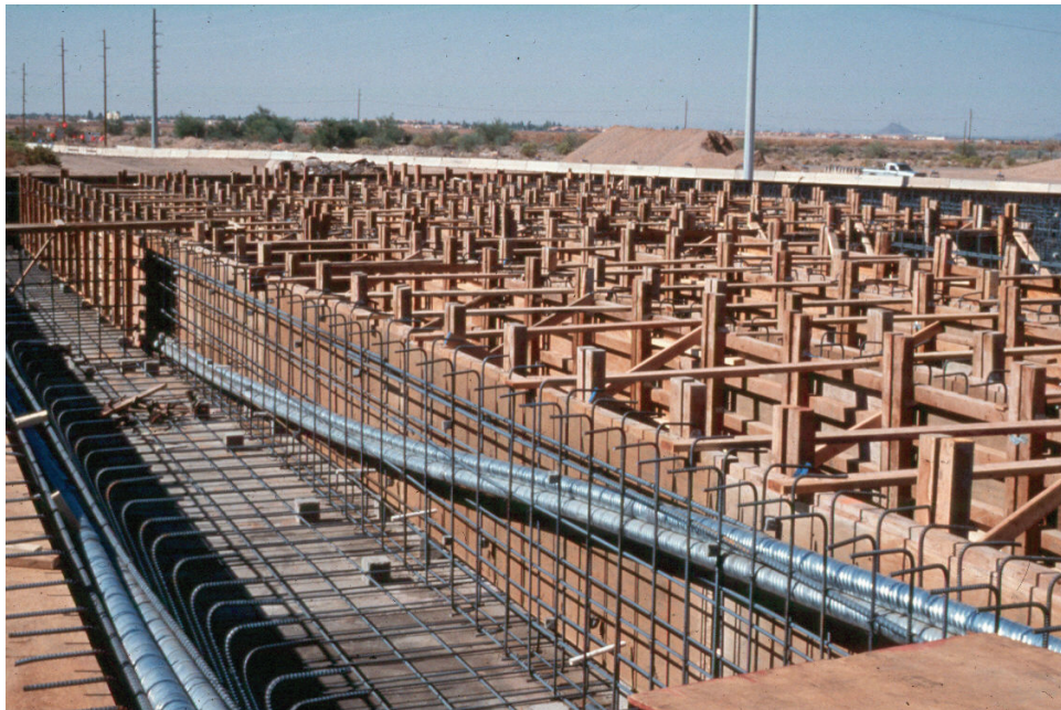
Figure 7.11.36 Post-tensioning Tendon Duct
