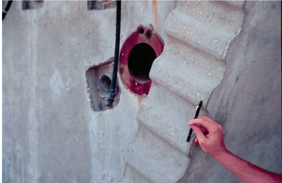
Figure 7.11.41 Close-up View of Box Girder Shear Keys
