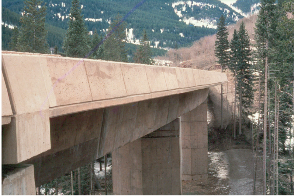
Figure 7.11.4 Cast-in-place Concrete Box Girder Bridge
