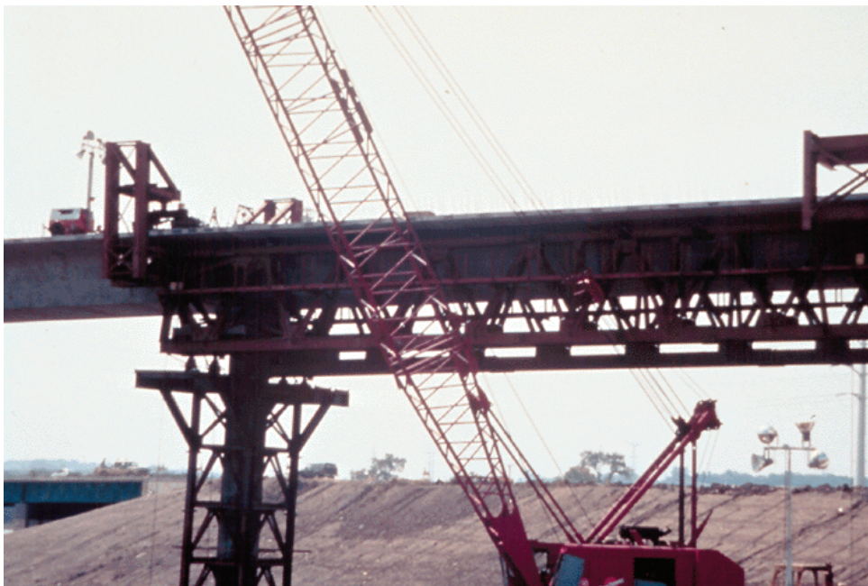
Figure 7.11.21 Span-by-span Close-up (with Erection Truss)
