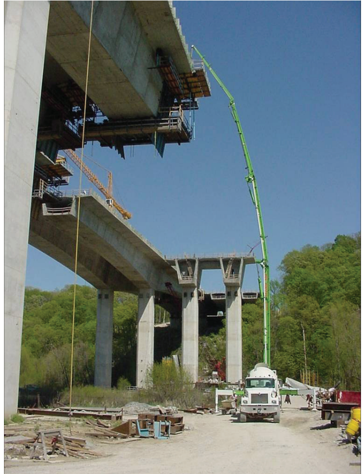
Figure 7.11.23 Progressive Placement Construction
