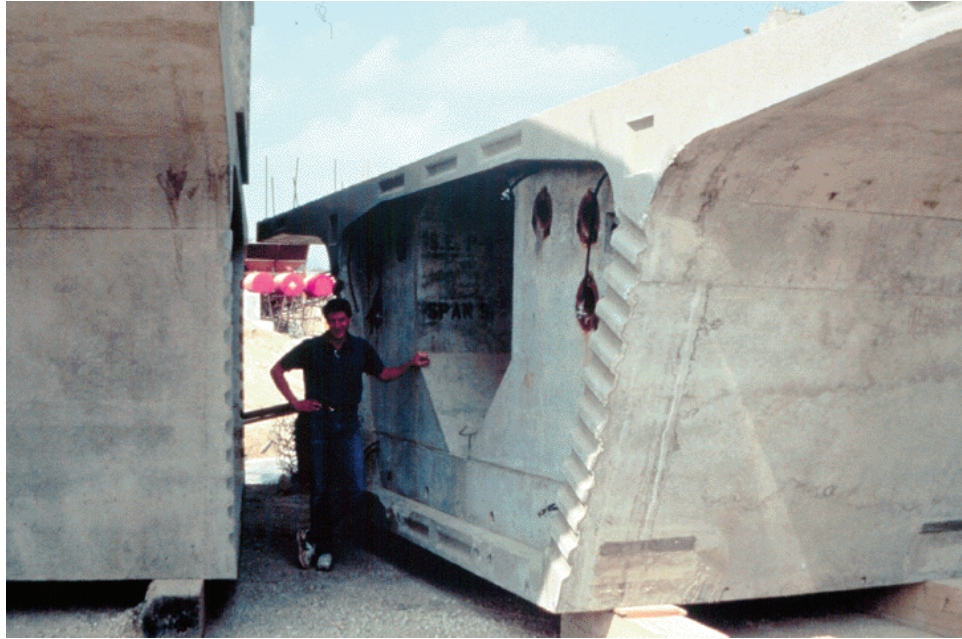
Figure 7.11.43 Box Girder Interior (End) Diaphragm
