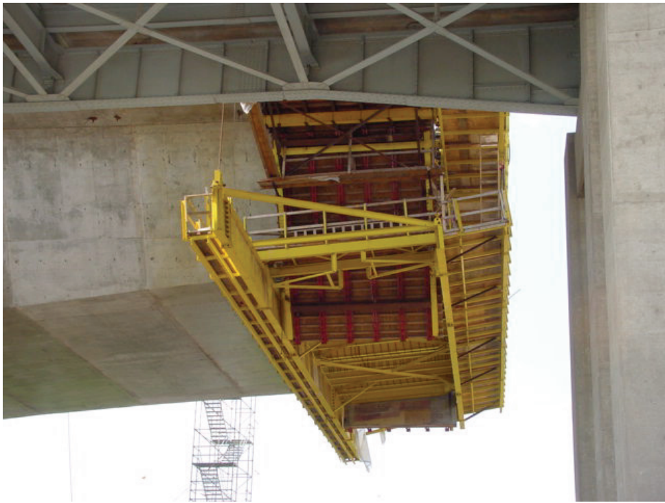
Figure 7.11.15 Cast-in-place Box Girder Segment
