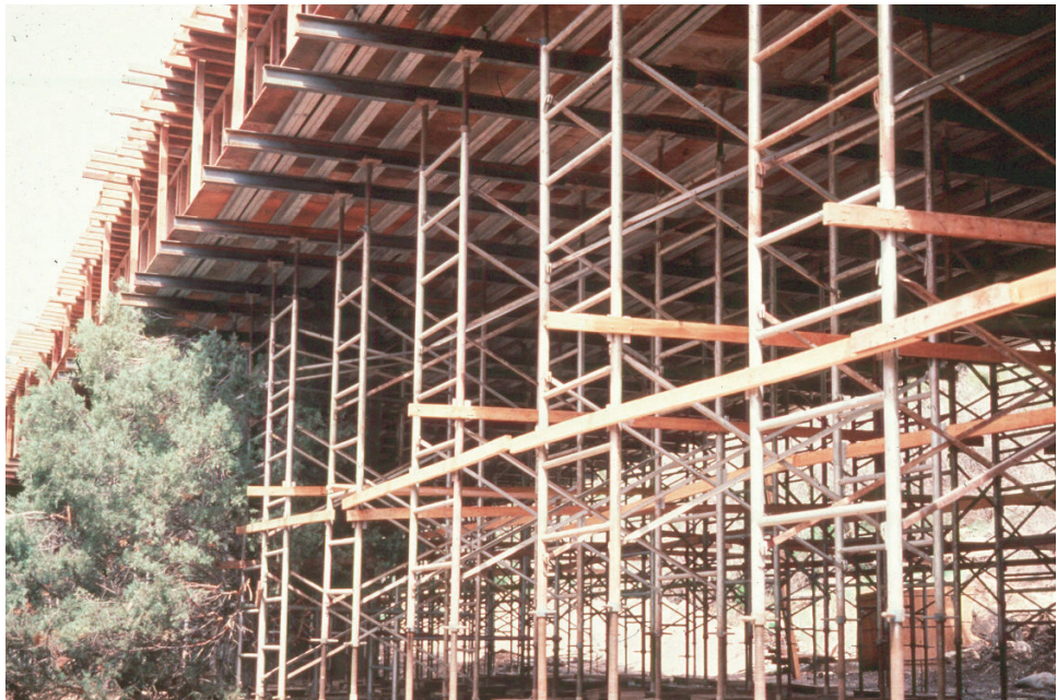
Figure 7.11.5 High Level Casting Formwork on Falsework
